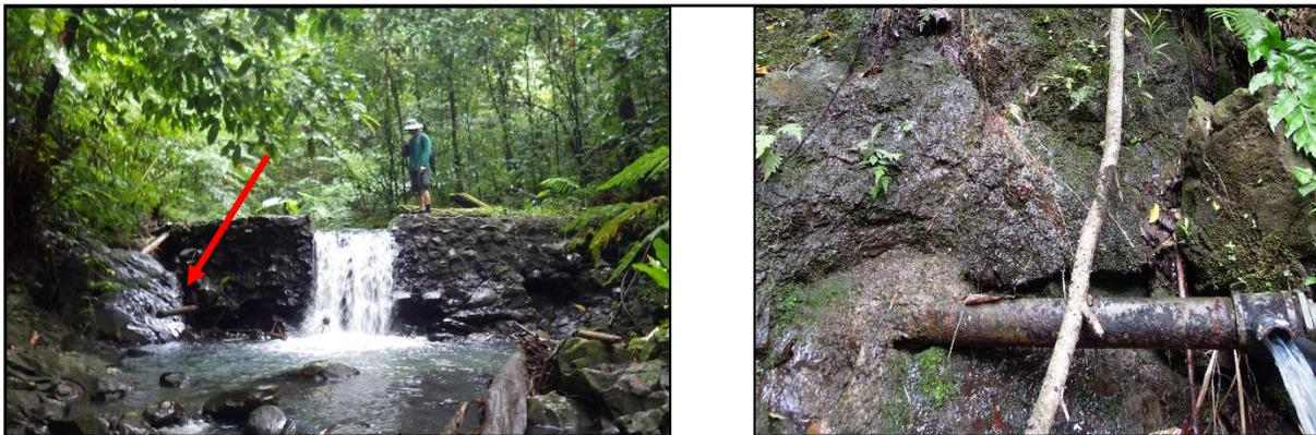
Figure 15: Example photos of village water system intakes. Abandoned village water impoundment across Fagaalu stream (left). Note old delivery pipe as indicated by red arrow. Village water intake located directly in volcanic spring in rock face of cliff in a village near Nuuuuli Village (right)
