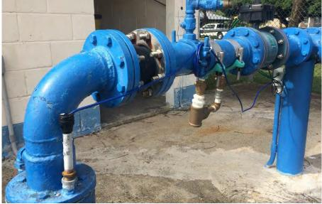
reduction and modulation of flow through the sensor. Well 62 has no well-pad riser, but the casing itself extends 62 cm off of the concrete well slab, and the top of the sounding tube stands about 20 cm above the casing top.
