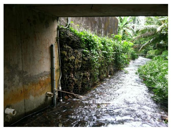
Control structure for Fagaalu gage, downstream channel control. April 2016
