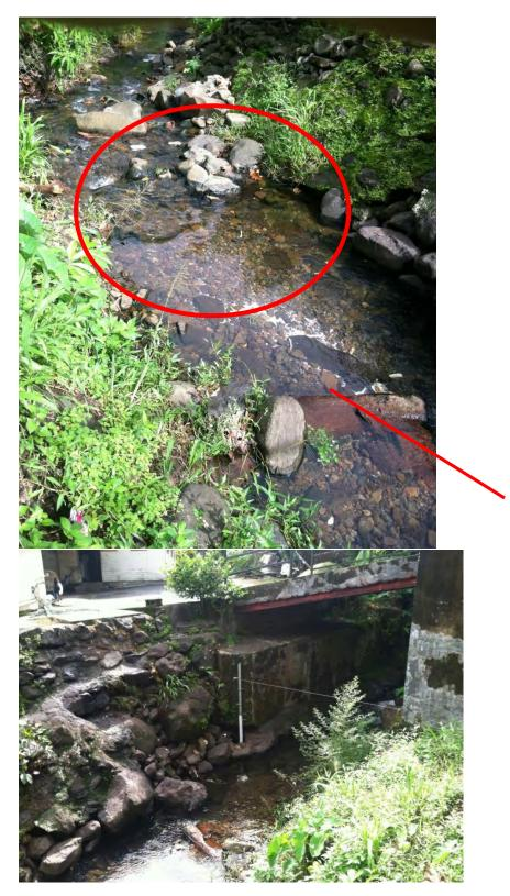
Control structure for Fagasa gage, rock bar in top center of top photo. Note position of red rock in both photos. April 2016
