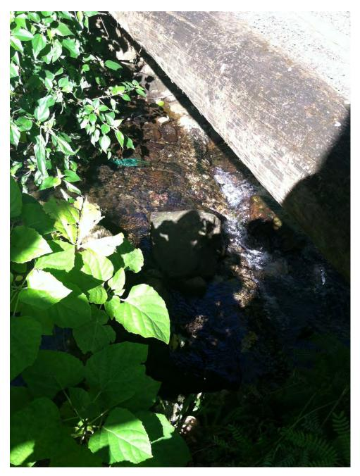
Terrible photo of control structure for Afono gage, shows old USGS concrete weir structure. Weir has a gap in the middle where a large boulder has lodged. April 2017
