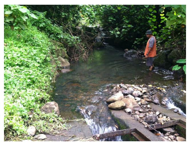
Control structure for Malota gage, rocks piled at culvert entrances. April 2016
